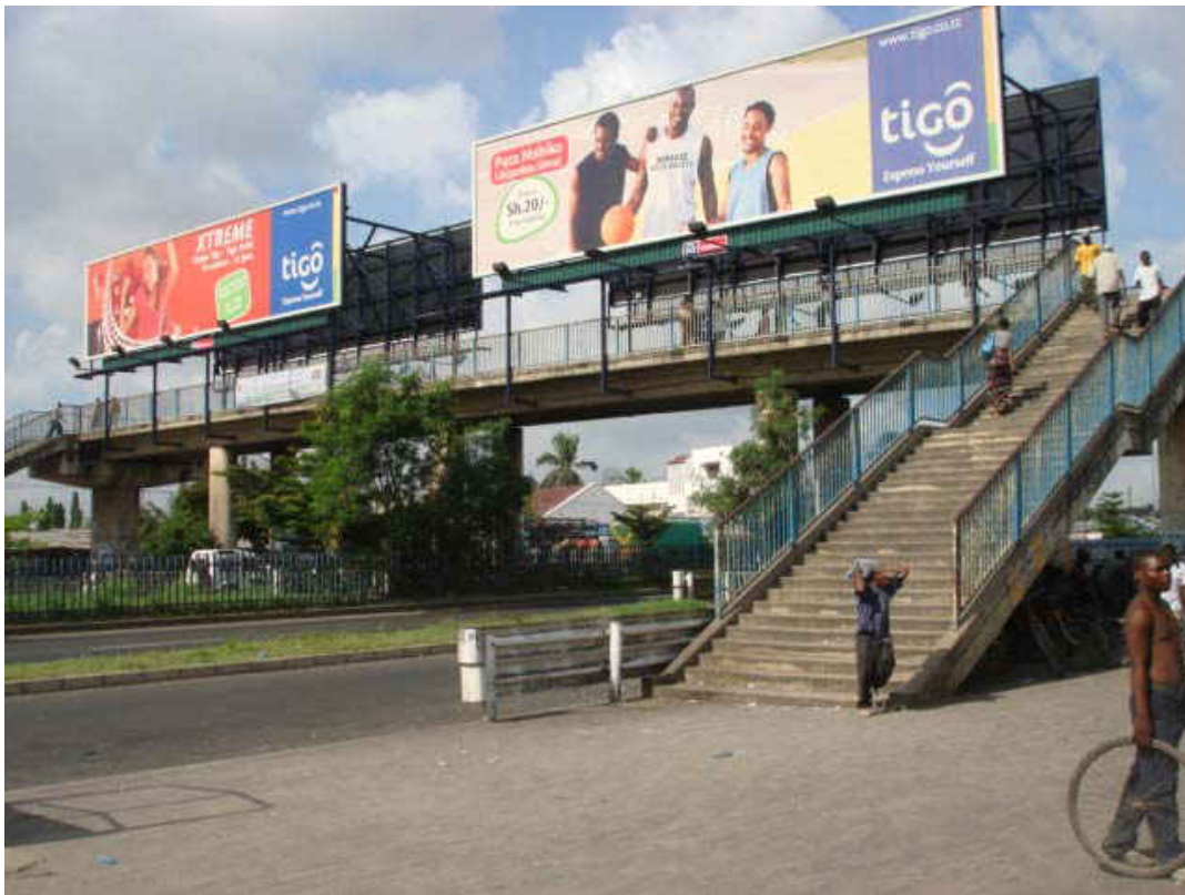
Figure 1. Manzese Foot Bridge
